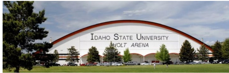
Conceived and developed by ISU athletic director Dubby Holt, the facility was renamed in honor in 1988.
